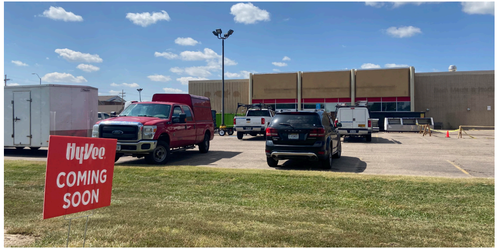
Remodeling has started on the new Holdrege Hy-Vee location on north Burlington Street. The store will employ 11 full-time and at least 34 part-time employees.
