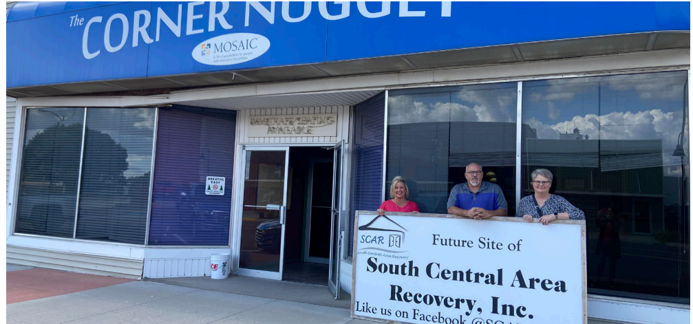
A PCDC GO! DREAM grant helped South Central Area Recovery replace a leaking roof in its new building this summer. Pictured are Board Members Gayleen Maurer, Dean Lynch and Carie Lynch in front of SCAR's new building that will continue to be remodeled over the winter.
