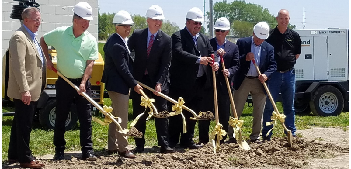
Gov. Pete Ricketts (fourth from left) attended the Allmand Inc. expansion groundbreaking in May.
